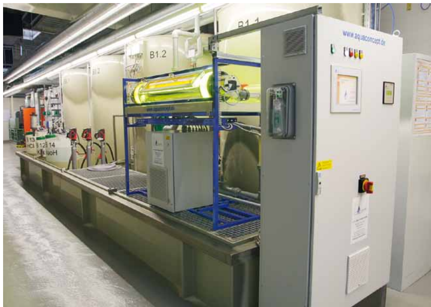
Fig. 4: Enviolet®-UV-Installation for 100% destruction of APIs.
