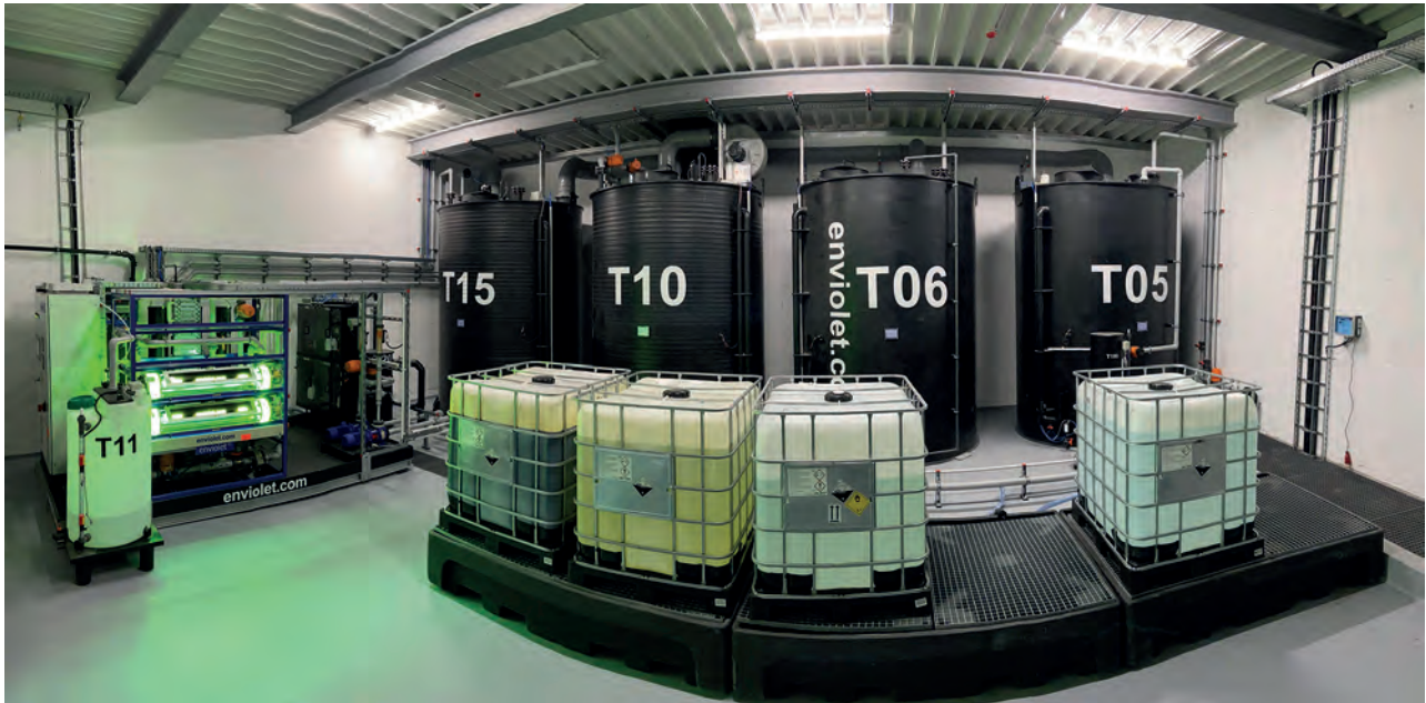
Figure 17: Batch treatment plant for about 20 m 3 /d pharmaceutical wastewater containing APIs and bio-active material.
