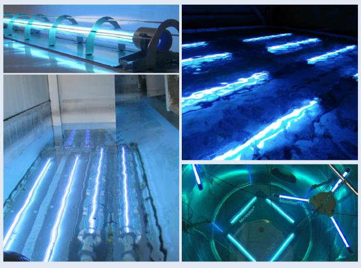
Figure 6: Cooling Tower with Installed UV-Lamps, Type Microfloat® & Microspear®
