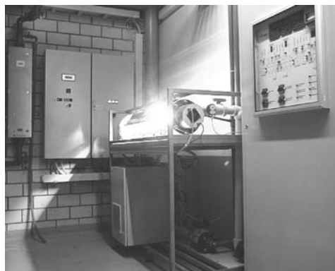
Fig. 2: Enviolet UV-reactor of CyanoMat®-system at FUBAG
